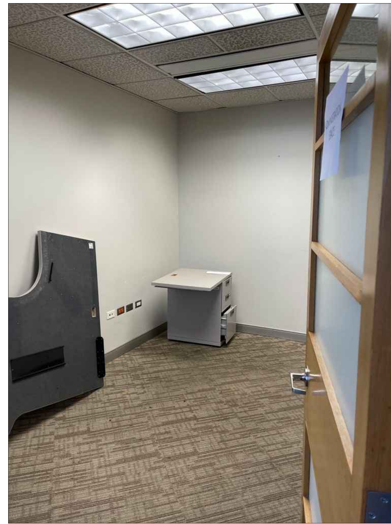
05 EXISTING CONDITION_POST PRODUCTION ROOM
